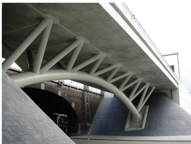
Figure 1. Merxem street tubular arch bridge
