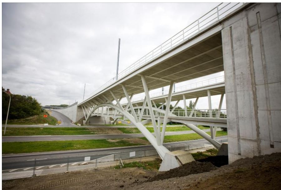
Figure 2. Woluwe Lane Bridge
