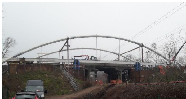
Figure 22. Bridge with temporary bracing
