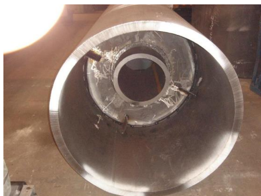
Figure 8. Fabrication of internal stiffening
