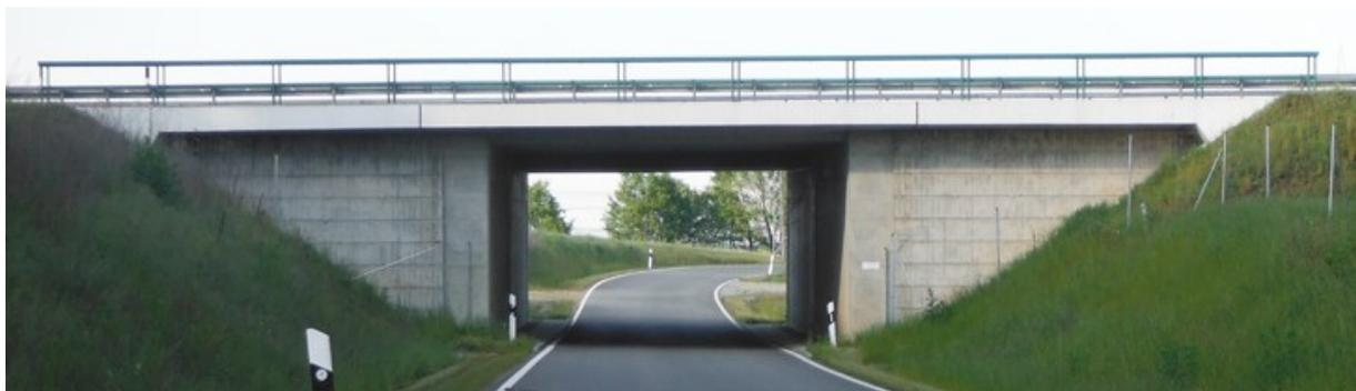
Figure 6. Single-span concrete slab bridge
