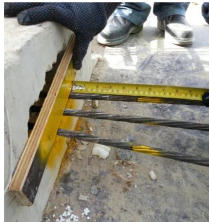
Figure 20. Mono strand stressing jack (left) and measurement of achieved elongations (right) (both obtained from Contractor's document Method Statement for Post-tensioning worksRS\_BW\_P19.1\_C\_025\_PZM\_MST\_0021\_Rev.00\_Post Tensioning Works)
