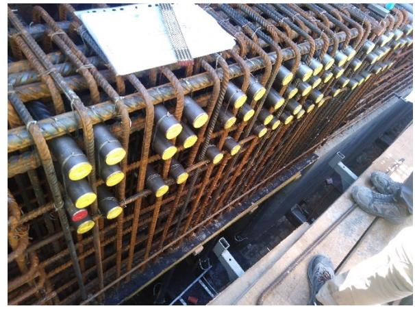
Figure 17. Lenton couplers for Transfer beam on Level 20 at core wall in Contractor's shop drawing (left) and on site (right)
