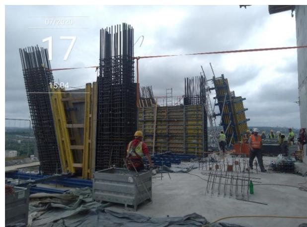
Figure 15. Construction of transfer branching columns Levels 14-15 (left) and Levels 15-16 (right)
