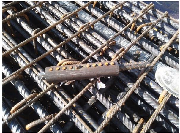
Figure 16. Transfer beams on Level 12 (top row) and on Level 20 (bottom row) – details of coupled bars (bottom left) and discarded coupler (bottom right)
