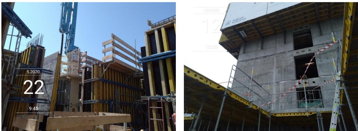
Figure 12. Construction of core walls in jump form
