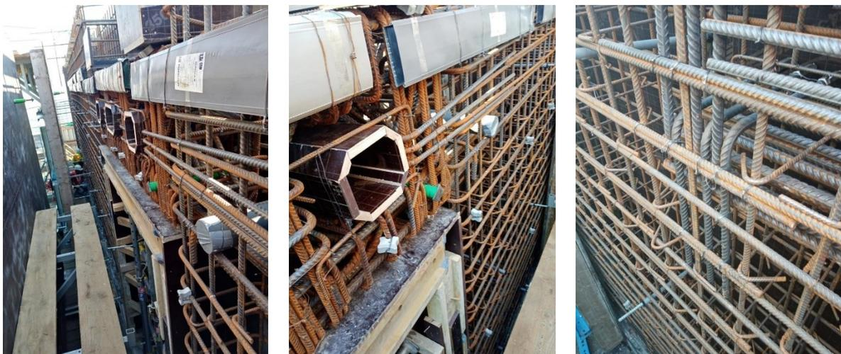
Figure 13. Link beam reinforcement with Bindax pullout boxes on top - installed into wall rebar cage (left and middle) and core wall reinforcement (right)
