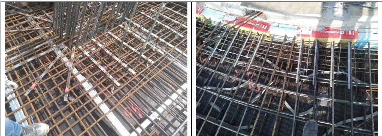
Figure 21. Halfen shear rails with double headed studs (left) and thermal connector at balcony location (right)
