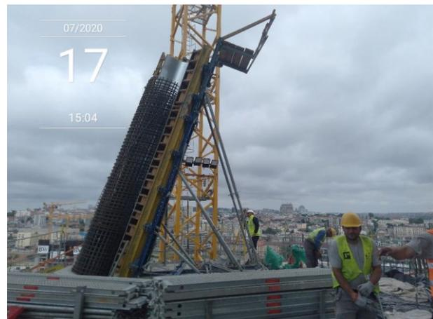
Figure 14. Construction of circular transfer columns Level 12-14 (left) and Level 16-17 (right)
