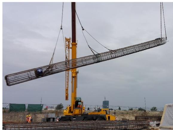
Figure 3. O-cell installed into the pile rebar cage (left) and insertion of rebar cage with O-cell into the borehole (right)
