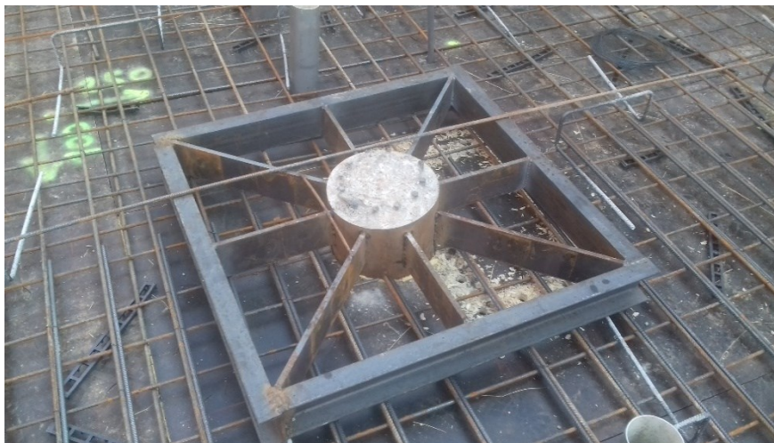
Figure 34. Steel structure for connection of piles and slab
