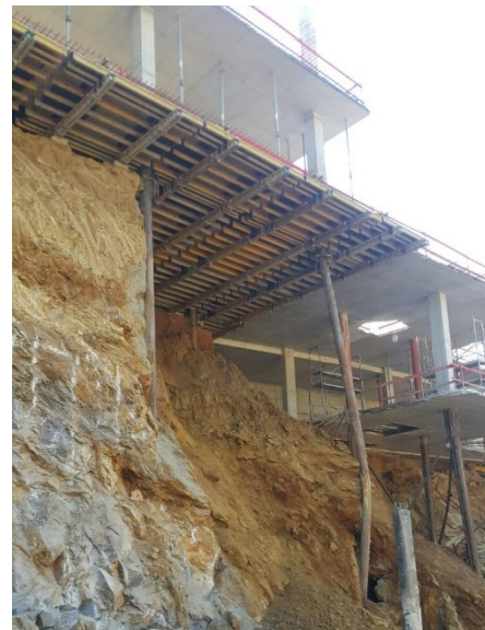
Figures 58 and 59. The failure of the steel column after the landslide. Steel column is bridged by a lattice steel structure placed on the slab above it. The load from the damaged column was transferred to the adjacent columns
