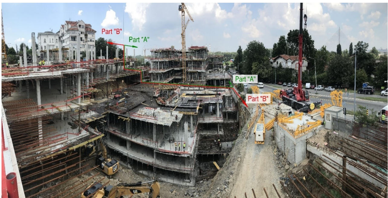
Figure 38. The first connection of the parts A and B was made with the third floor slab
