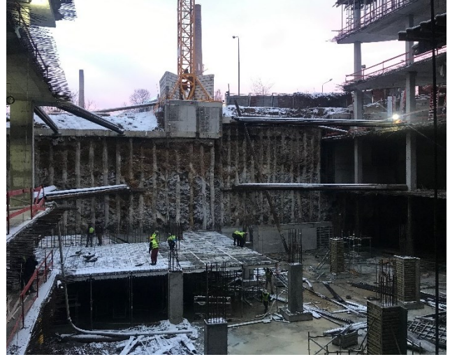
Figure 48. Temporary ramp is cancelled. Mechanization from Visoka Street passes under the building to Radnicka street going outside
