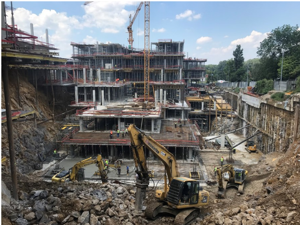
Figure 26. Part A of the building under construction in an advanced phase
