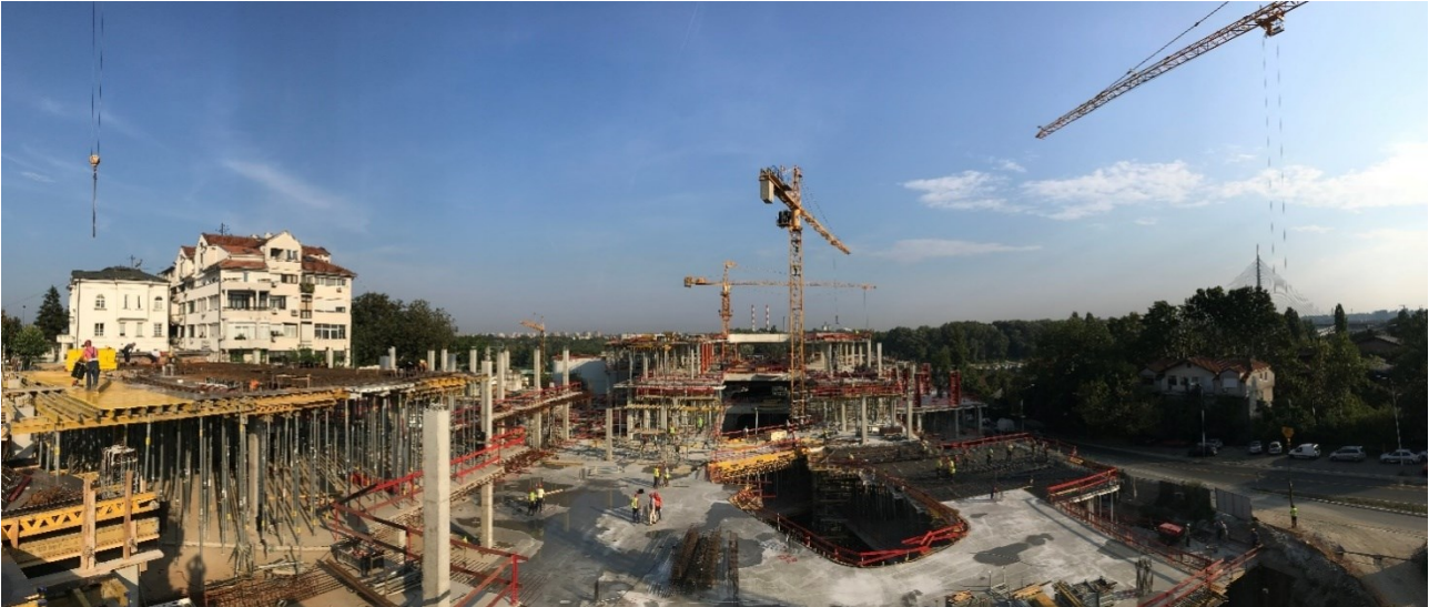
Figure 50. Unobstructed construction of the last floors while the top down works are performed in the underground
