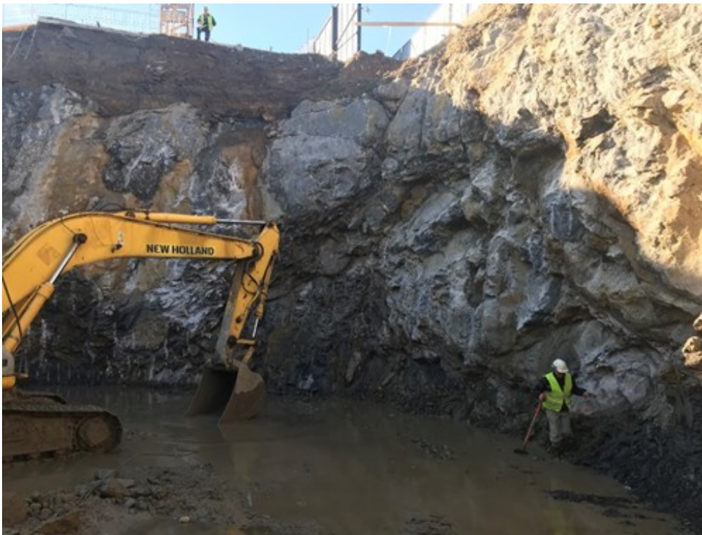
Figure 24. Extremely strong rock zone where vertical excavation was done without protection
