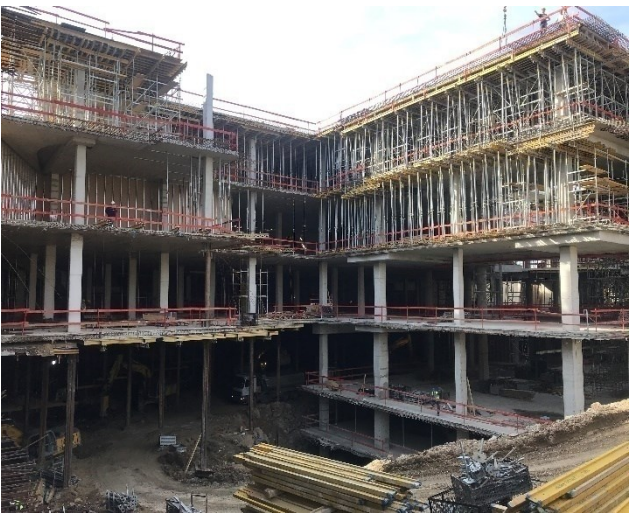
Figure 49. Passage of machinery under the building and exit to the ramp along Radnička Street
