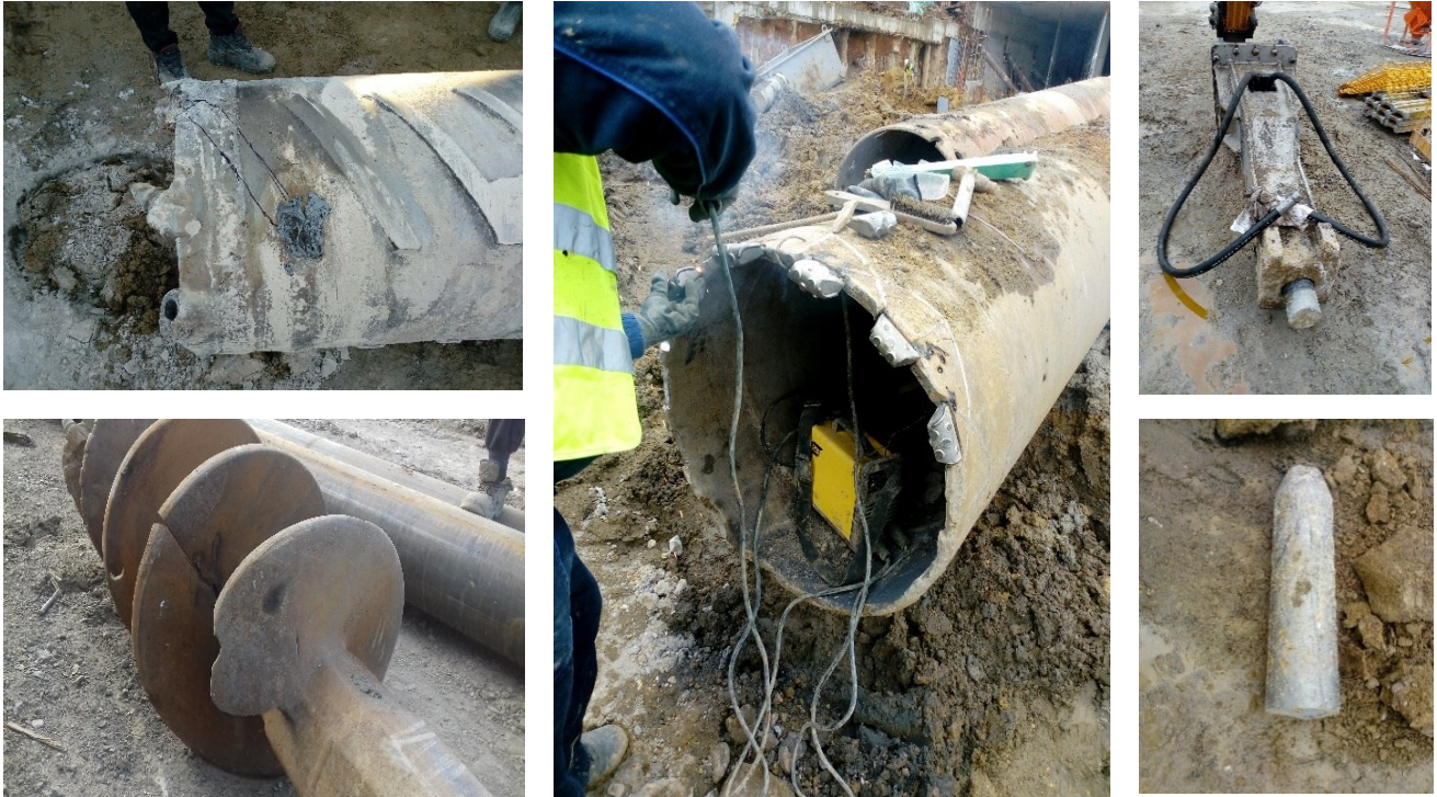
Figures 17-21. Broken drilling rigs, diamond teeth on the ranger and the spikes of a hydraulic hammer
