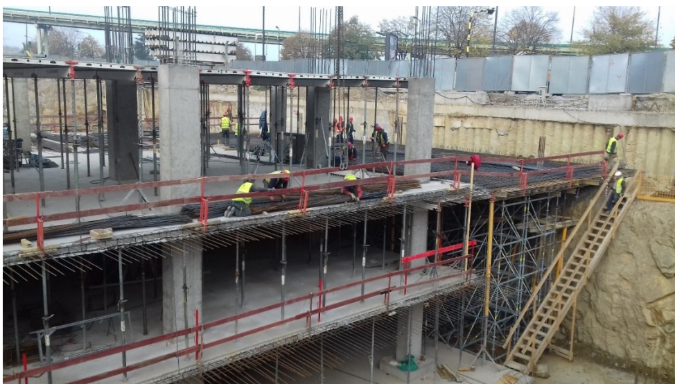
Figure 14. Strutting by -1B slab over the berm (the slab is supported by temporary steel frame and steel pile (future RC columns))
