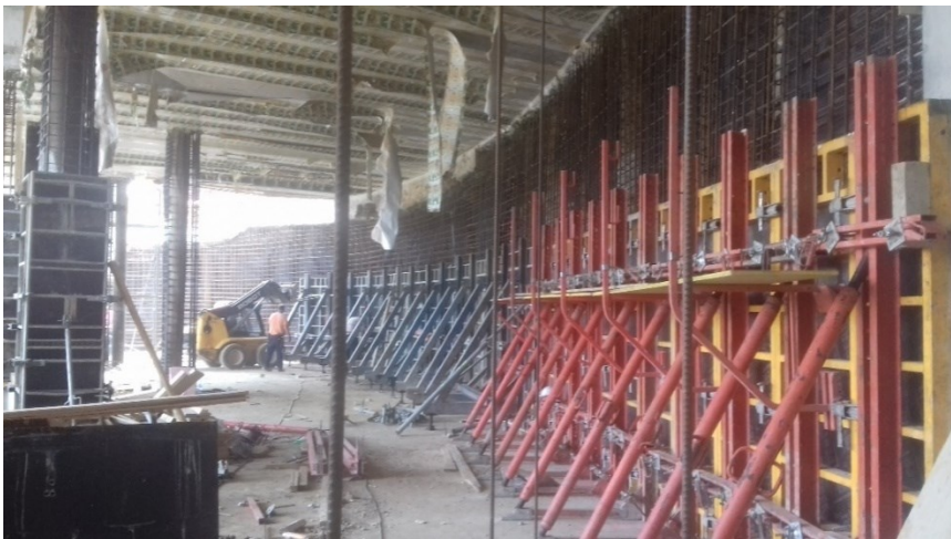
Figure 43. Shutter erection of formwork of the perimeter wall - formwork with one-sided formwork
