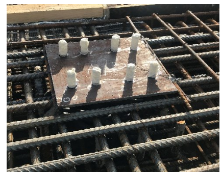
Figure 54. Anchor plate for steel column
