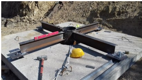
Figure 29. Concrete platform with steel guide
