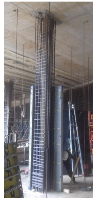
Figure 44. Column reinforcement installing around the steel pipe of the pile
