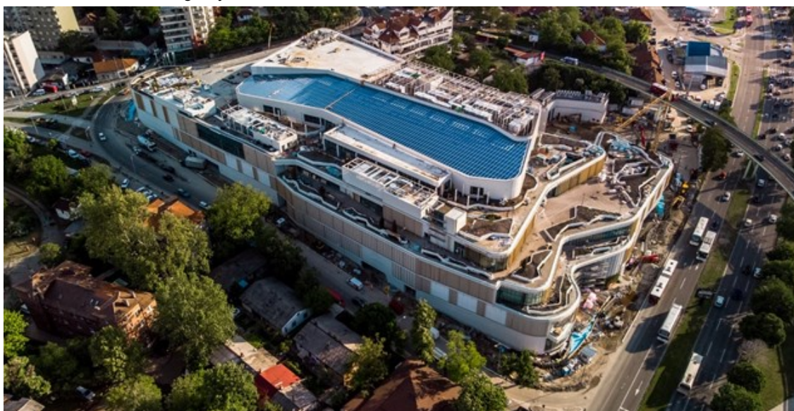
Figure 1. Shopping Center Ada Mall under construction
