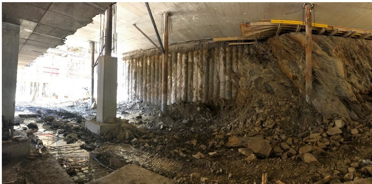
Figure 16. Excavation of the berm under finished structure. Secant piles, temporary steel columns (piles), formwork installed at the berm
