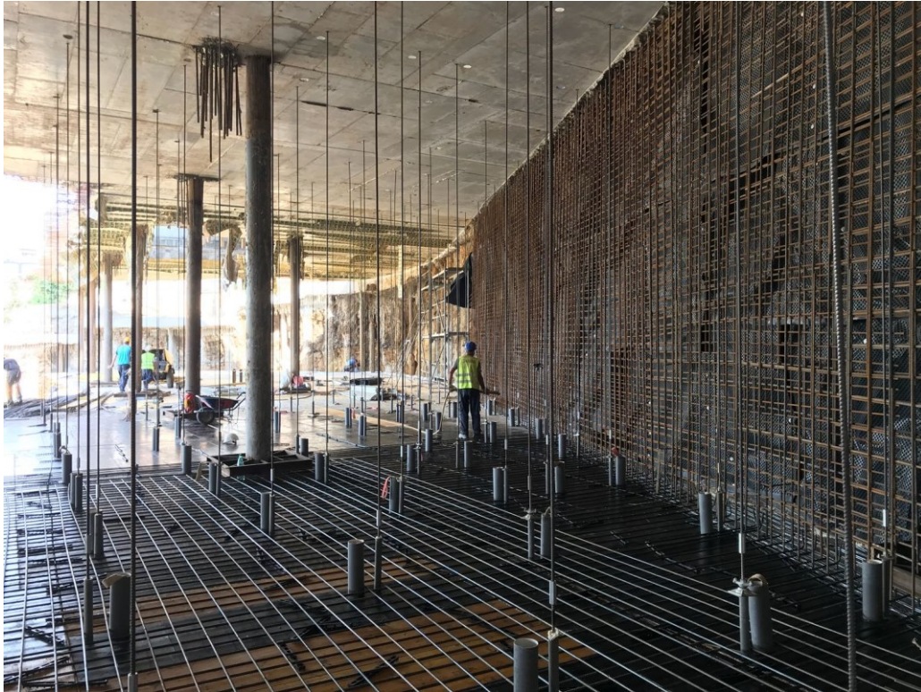
Figure 42. One of the hunged slab in the top-down phase (part B, zone 2)
