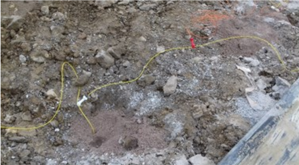
Figure 23. The explosive was inserted into the holes and interconnected with decelerators
