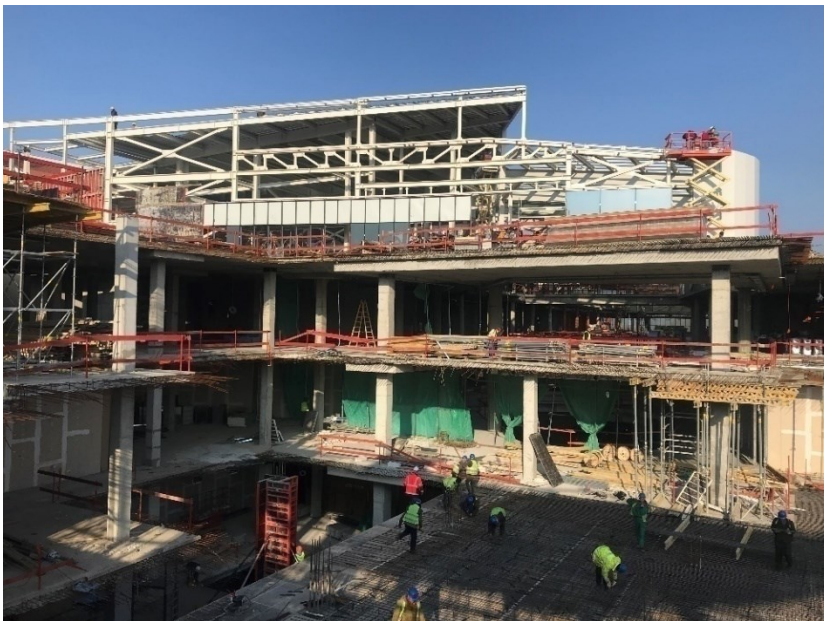
Figure 53. The construction of steel and concrete structure in parallel
