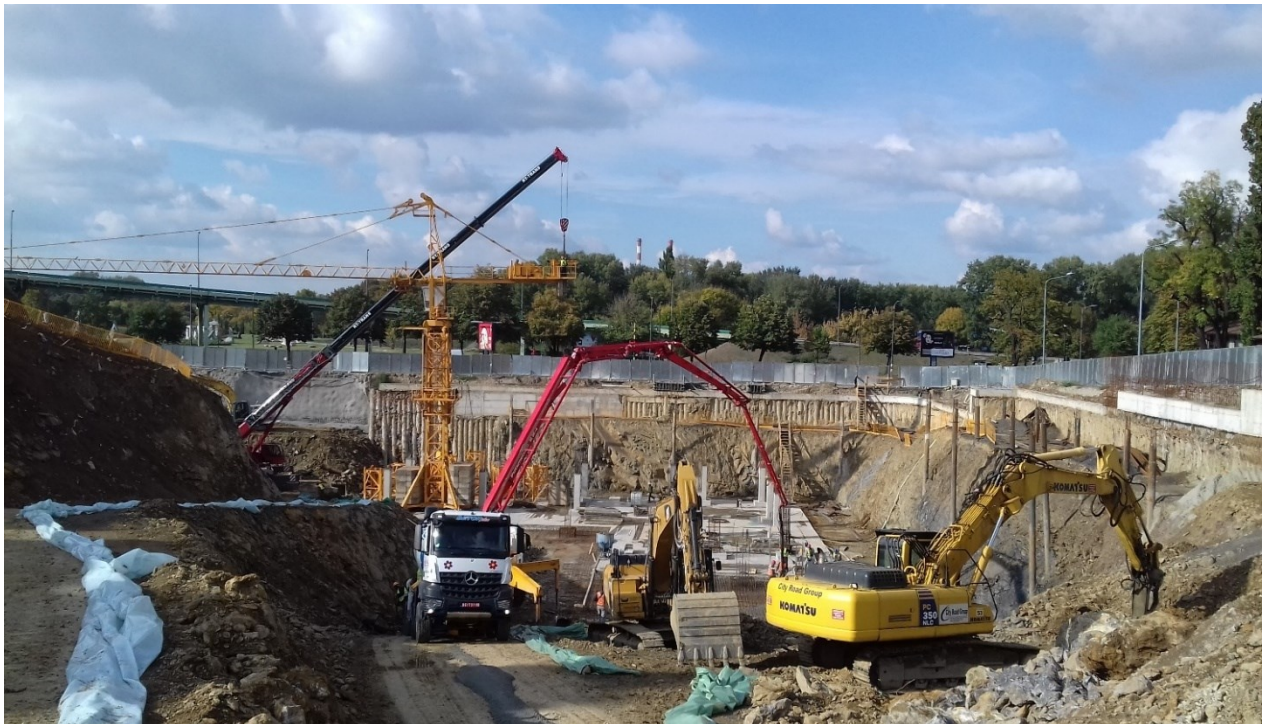
Figure 11. Part A wide excavation with formed berm (zone 1) where piles were drilled at the column locations
