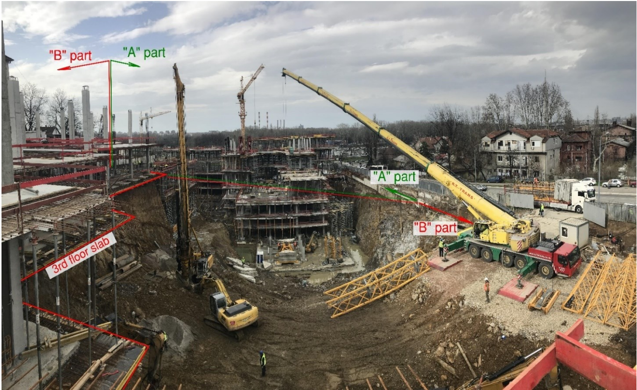
Figure 35 .Part A is in an advanced phase and is progressing towards part B where the construction started from the 3rd floor upwards
