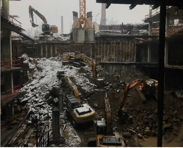
Figure 47. Cancellation of the temporary exit ramp
