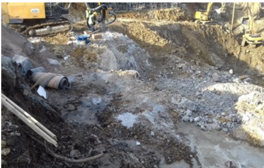
Figure 22. Drilling a hole for explosives
