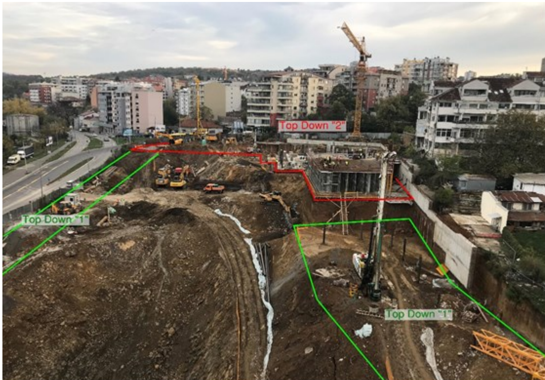
Figure 28. Construction of part B, Top Down 2
