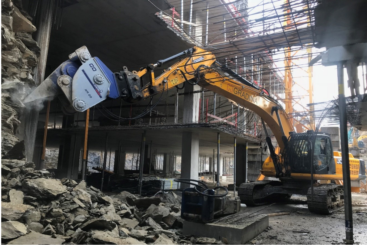
Figure 15. Excavation of the berm under finished structure with hydraulic hammers and rippers
