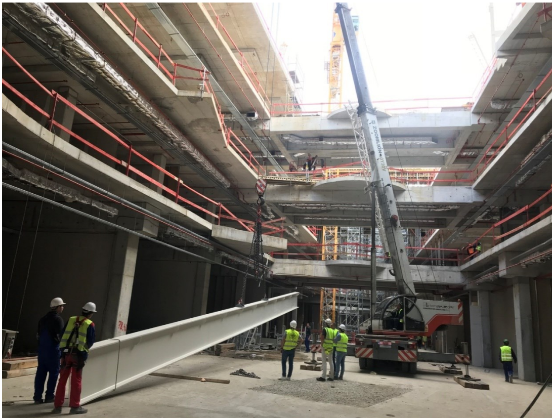
Figure 51. Installation of the steel roof structure from the atrium zone of the ground floor slab
