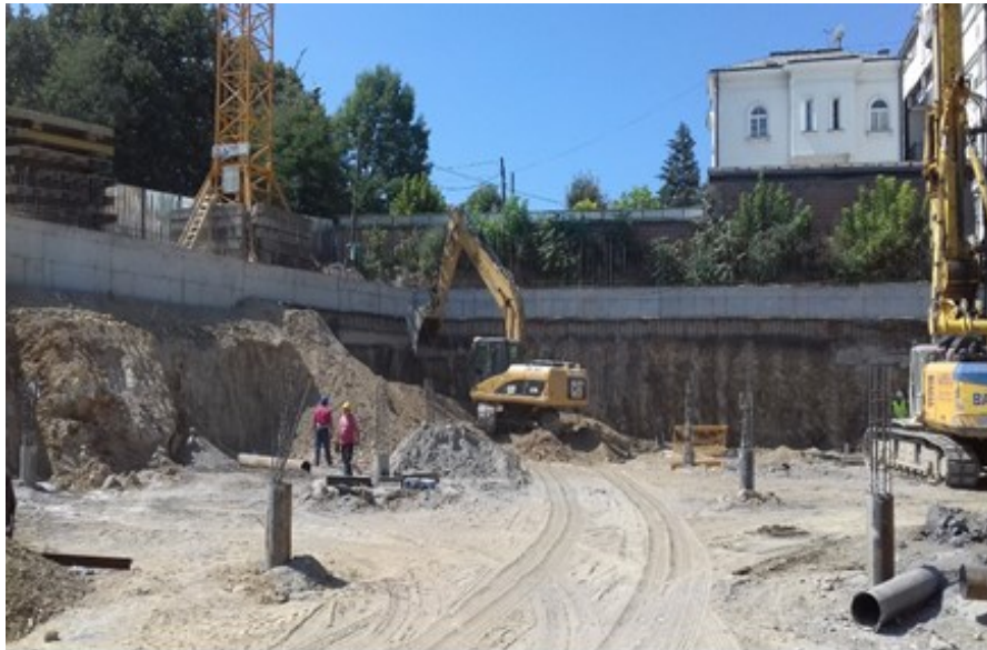
Figure 27. Construction of part B, zone 2
