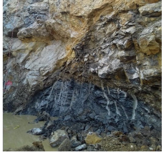
Figure 55. Different layer of the bad soil in the rock mass
