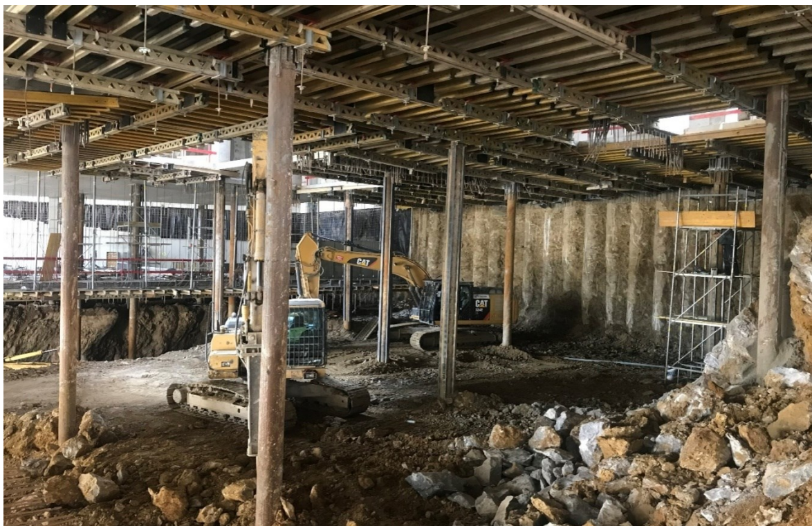
Figure 40. Excavation in the top-down phase below the constructed part of the building (part B, zone 2)
