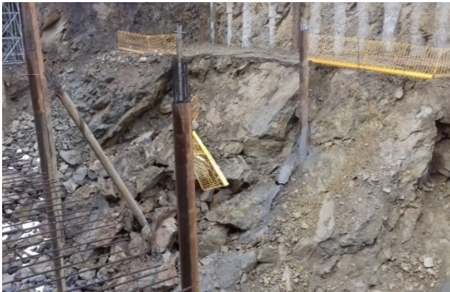
Figures 56 and 57. Damaged steel columns due to a local landslide
