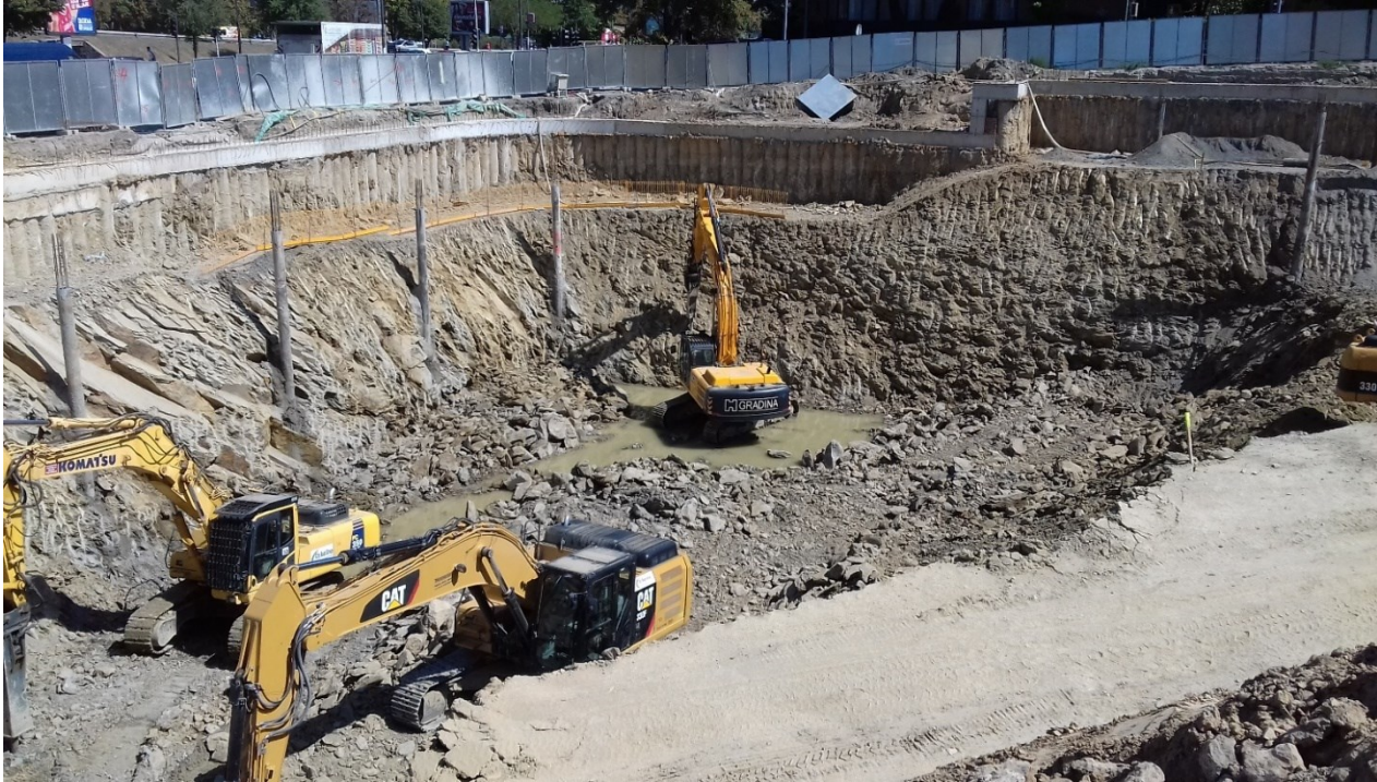
Figure 10. Part A wide excavation (up to the depth of 12 m) with the formation of a berm (zone 1) where piles were drilled at the column locations
