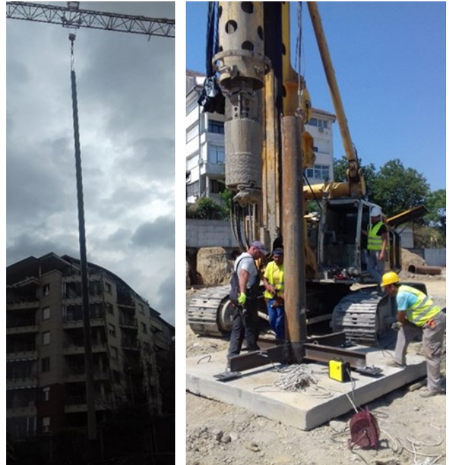
Figures 30 and 31. Installation of the steel pile through the "guide" for pile installation
