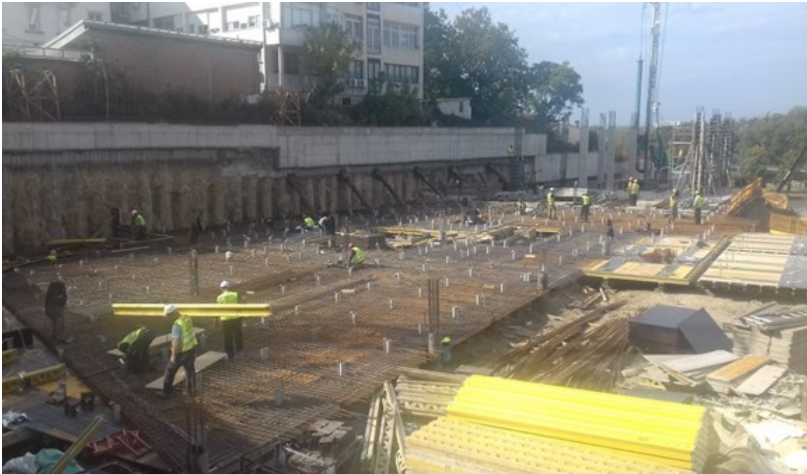
Figure 33. Installation of formwork tables of the third-floor slab on the ground (Part B, zone 2)
