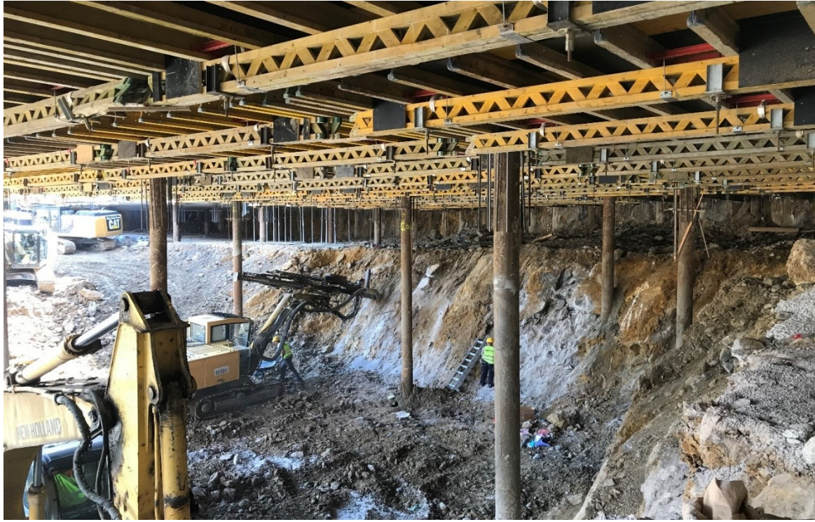
Figure 39. Blasting under formwork tables and the third floor slab (part B, zone 2)
