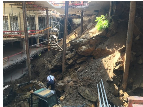
Figures 56 and 57. Damaged steel columns due to a local landslide
