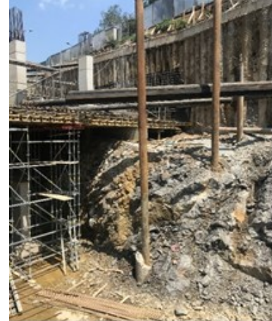
Figure 12. Installed formwork at the surface of the berm
