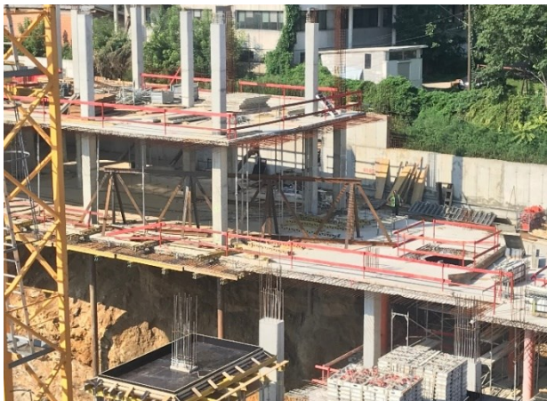
Figures 58 and 59. The failure of the steel column after the landslide. Steel column is bridged by a lattice steel structure placed on the slab above it. The load from the damaged column was transferred to the adjacent columns
