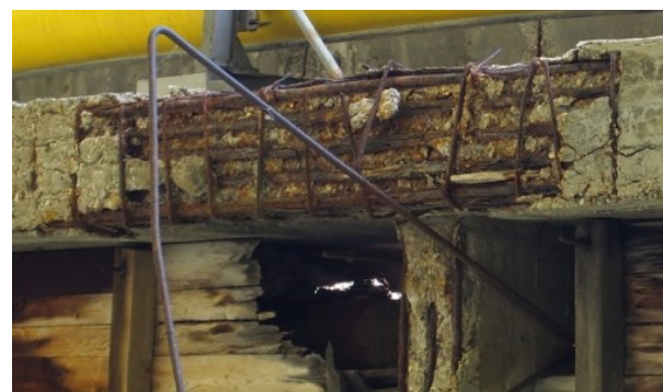
Figure 3. Severe corrosion of reinforcement, broken stirrups, deep spalling off of concrete, longitudinal girder in axis "C"
