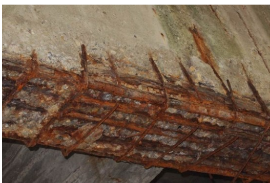
Figure 2. Severe corrosion of reinforcement, broken stirrups, longitudinal girder in axis "A"
