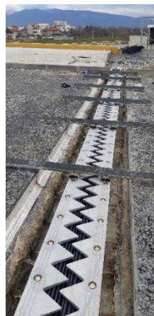
Fig. 5. Detail of an abutment, carriageway and sidewalk expansion joint
