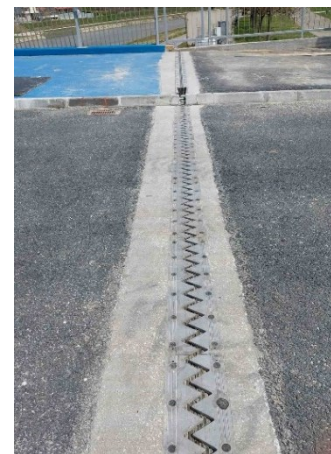
Fig. 5. Detail of an abutment, carriageway and sidewalk expansion joint
