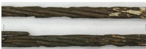
Slika 2. Kablovi koji su korodirali pre upotrebe, prema (Rinaldi et al, 2010) Figure 2. Cables corroded before their use, according to [7]
