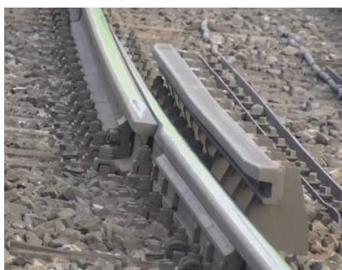
Slika 12. Diskontinuitet vozne površi u zoni dilatacione sprave Figure 12. Discontinuity of the running surface of the rail head at the expansion joint
